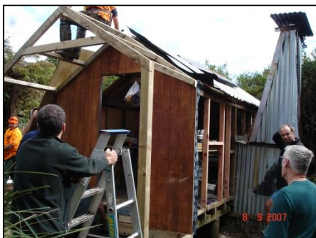
Rebuilding the Mangamuka Hut 2007 Kaimai Forest Park
