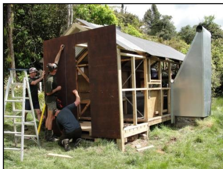
Rebuilding the Hurunui Hut 2010 Kaimai Forest Park
